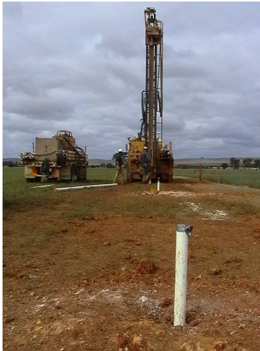
Figure 4: Nested piezometer construction
